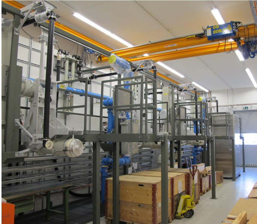
Installation of transmission line for new final stages
