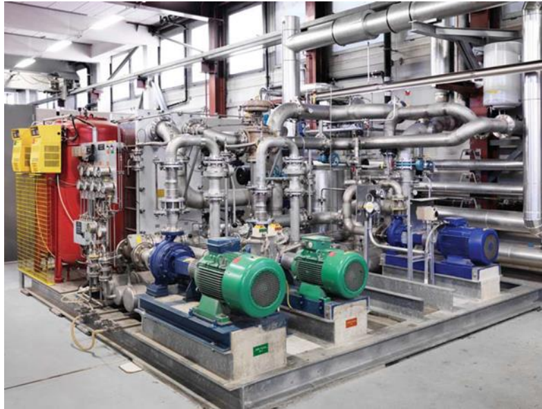
Cooling circuit HF0 for tetrode amplifiers for the ring cyclotron
