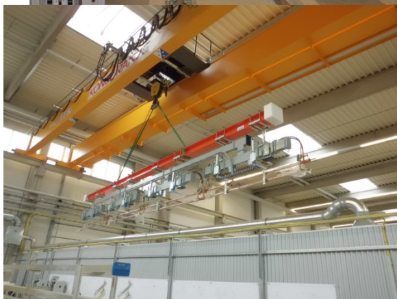
■ Waveguides at girder during installation test
