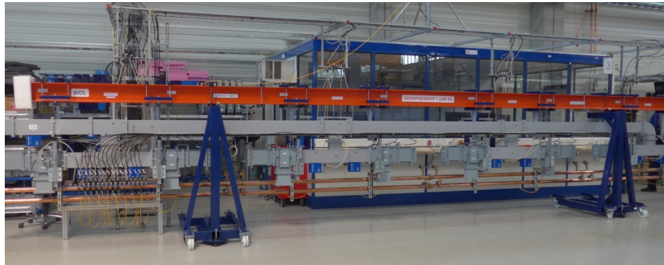
LLRF waveguide distribution test and tuning at WATF
