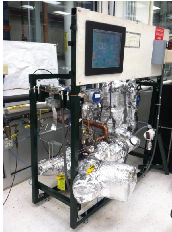
CO 2 cooling plant at FNAL
