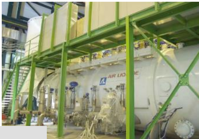
4.5 K refrigerators (18 kW @ 4.5 K)
