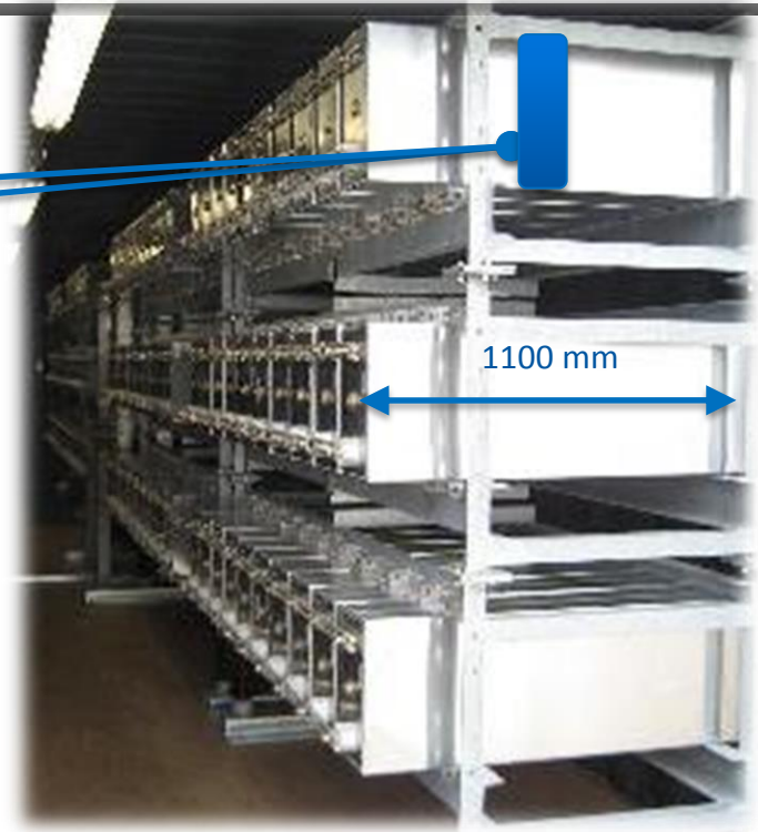
POPS capacitor bank at CERN. 6 Containers 65 tons
