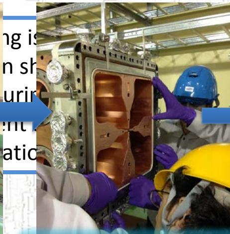
SM1-SM2 connection preparation
