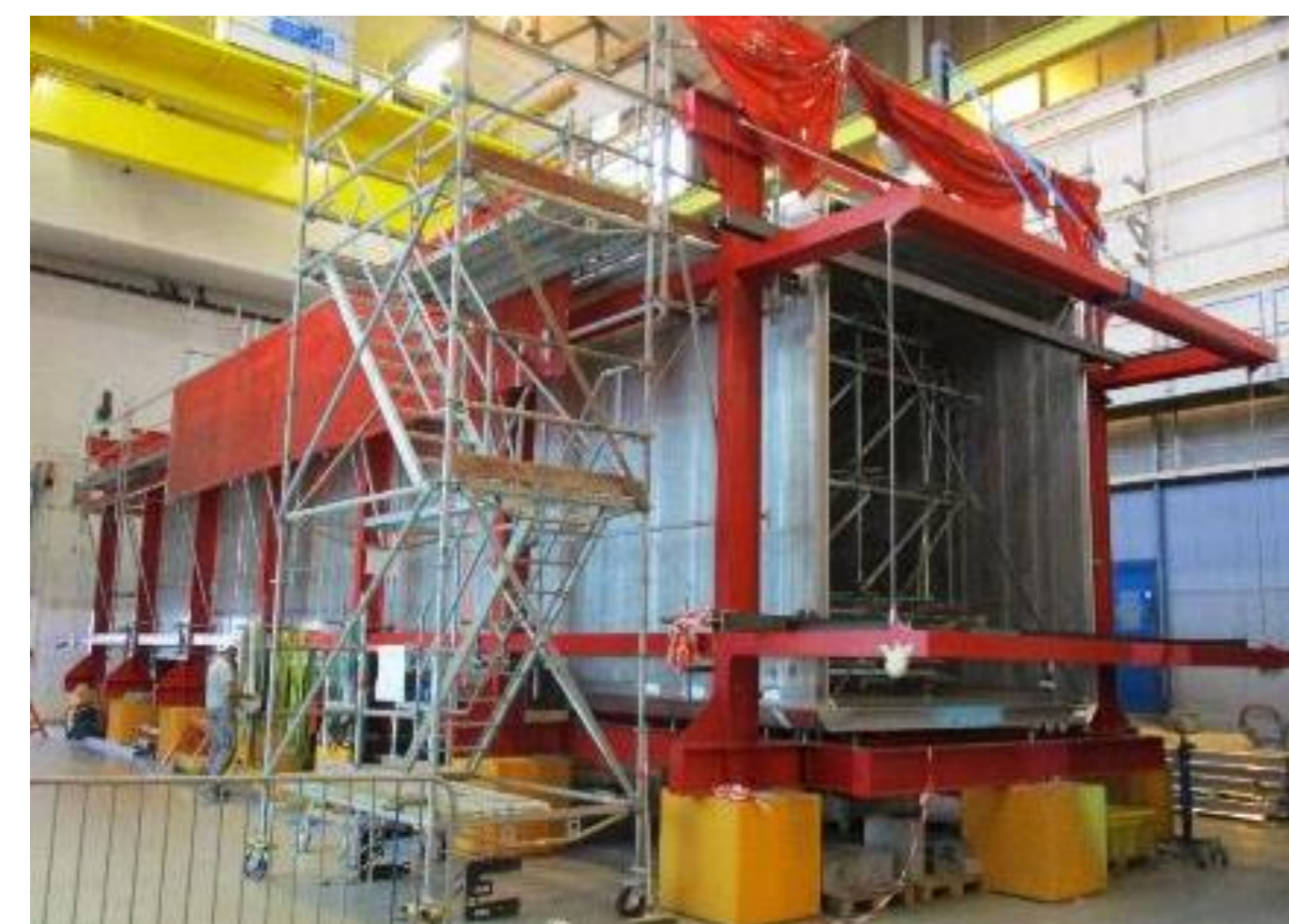
First WA104 cryostat under construction
