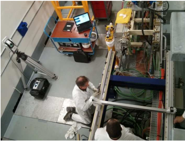
Figure 18: guide and support rails adjustments with MAT and laser tracker AT401
