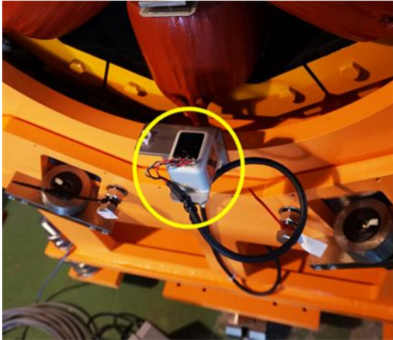
Figure 5: An inclinometer, enclosed within a yellow circle, is installed on the front face of the tilting table.
