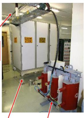
60kV platform for power converters Powered by Isolated 400VAC transformer 60kV Isolation 400VAC transformer
