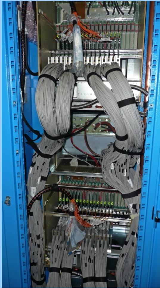
LVDS cables to Processors on backside of Preprocessor
