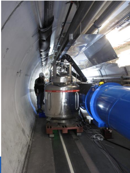
Helium dewars in place connected to the spill point. Dewars are pressurized by warm helium gas.
