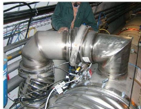
Damage to "jumper" connections of cryogenic distribution line
