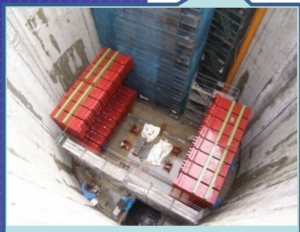
UA1 magnet donated From CERN installed
