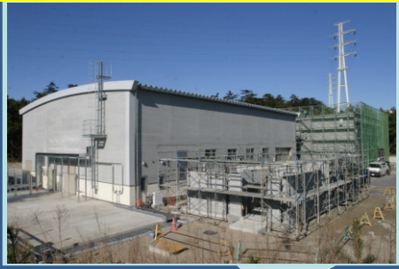
Neutrino monitor building
