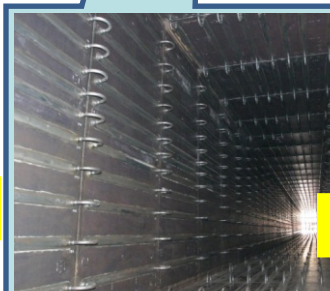
Decay volume completed
