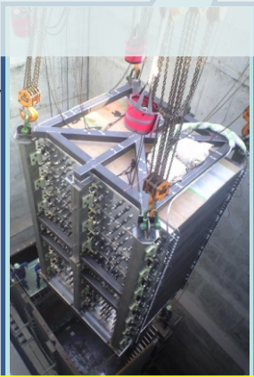
Beam dump installed
