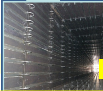
Decay volume completed
