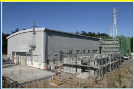
Neutrino monitor building
