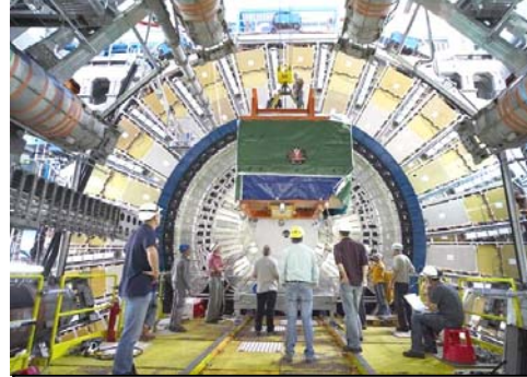
ID endcaps installed
