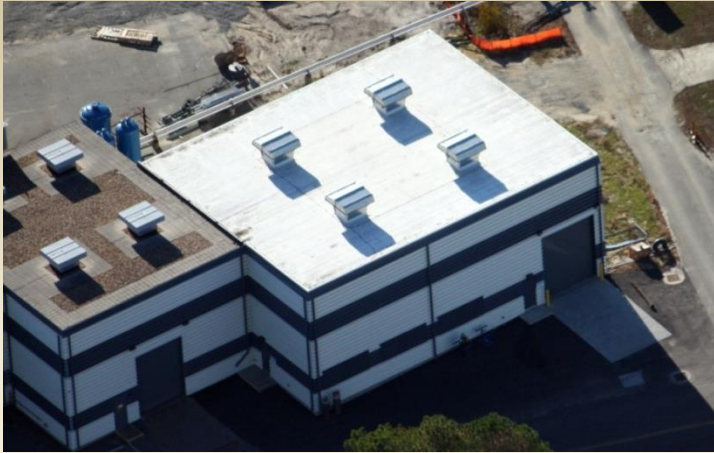
CHL Building Addition
