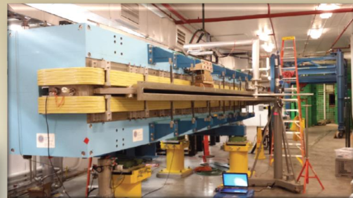
Hall D Tagger Magnet/Dump
