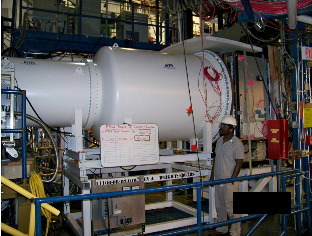
2-stage vacuum box in Hall B beam line
