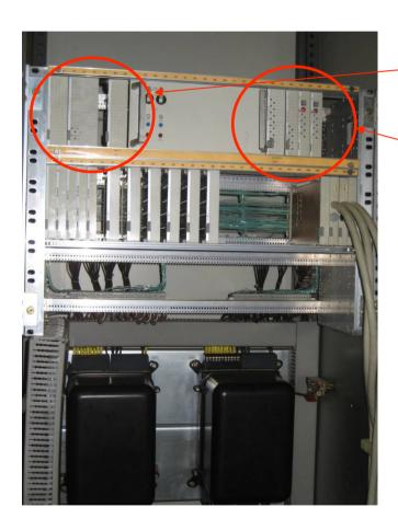
+/-15V Auxiliary Power Supply faulty
