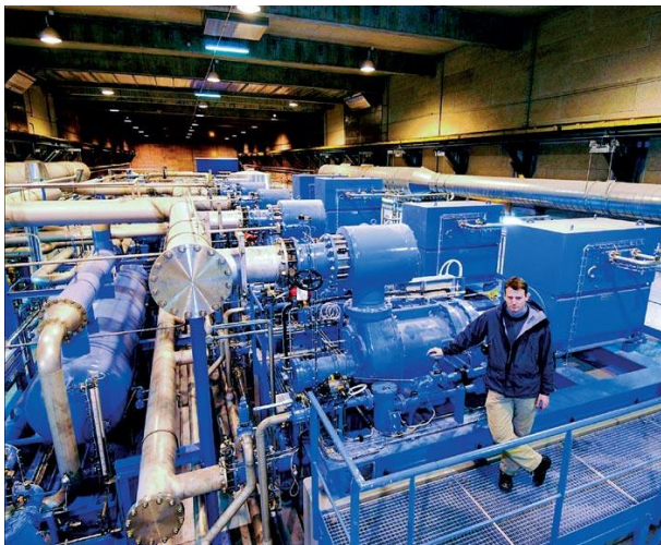
LHC compressors 18 kW @ 4.5 K
