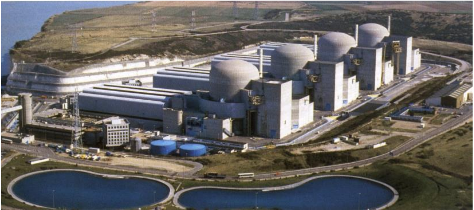
Paluel (F) Nuclear Power Plant 5.5 GW
