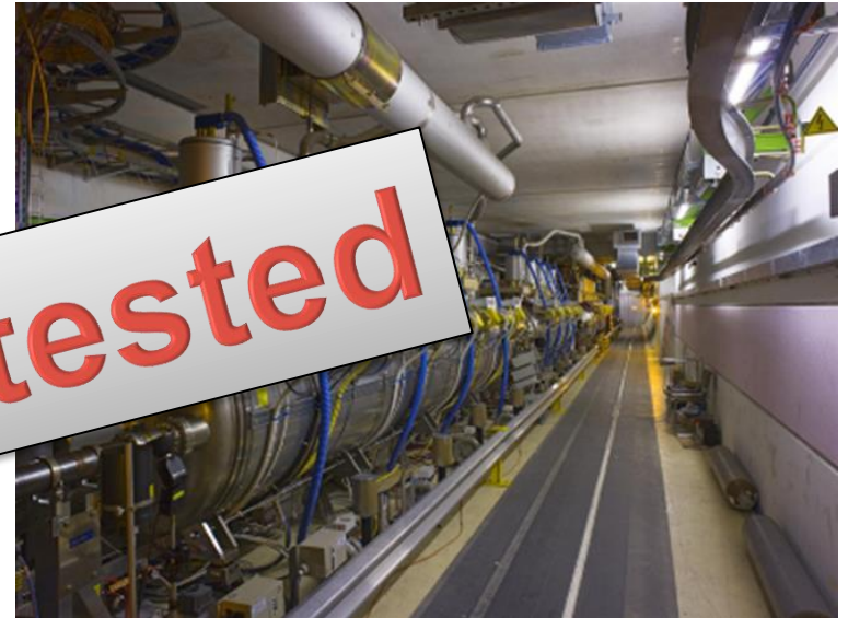
The Betatron Collimation System (250m long, 44 collimators + absorbers)
