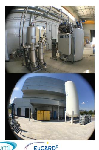
Our choice was a Linde LR280 with a 196 kW screw compressor. The procurement included the SFC for the compressor, a J-T liquid port, internal purifier, internal 80 K adsorber, He subcooler for single phase stream at 4.6 K up to 7 bar. Max 4.6 K flow is about 18 g/s.
