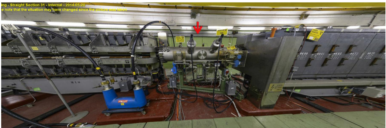
Figure 3.3: Straight section 31 overview.
