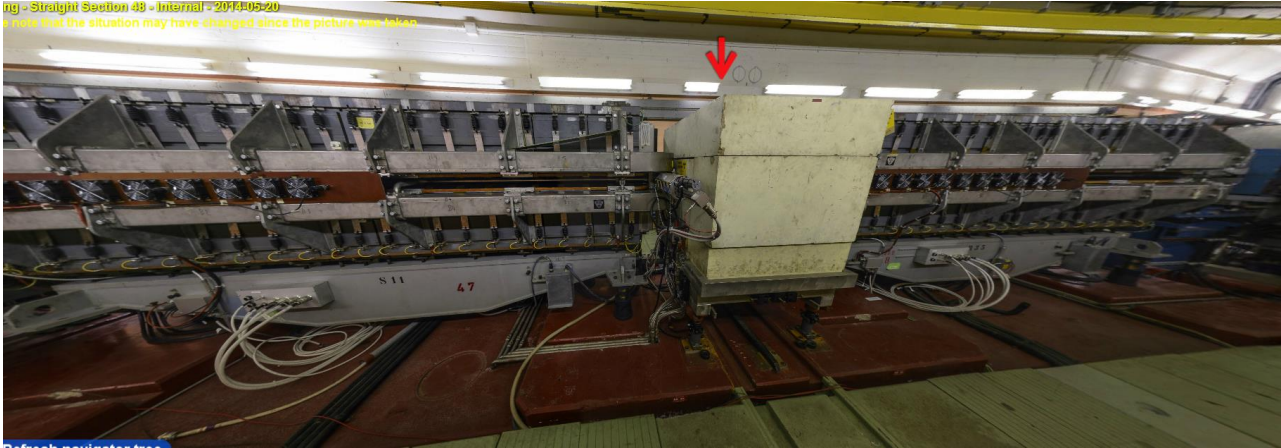
Figure 3.5: Straight section 48 overview.
