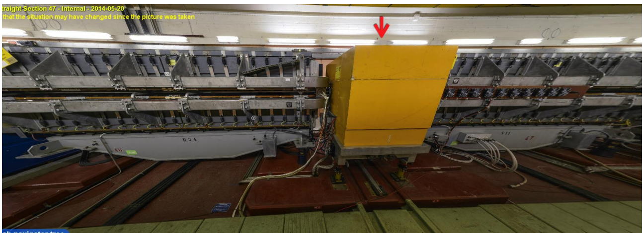
Figure 3.4: Straight section 47 overview.
