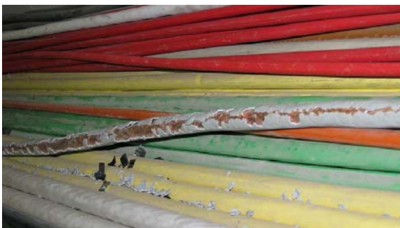
In the SPS tunnel:
