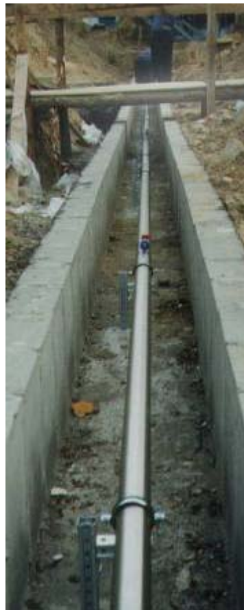
Liquid nitrogen and liquid helium transfer lines
