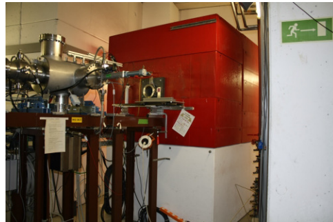
Beam dump for SIS18 synchrotron at GSI (made of iron 3×2×3 m with concrete shielding)
