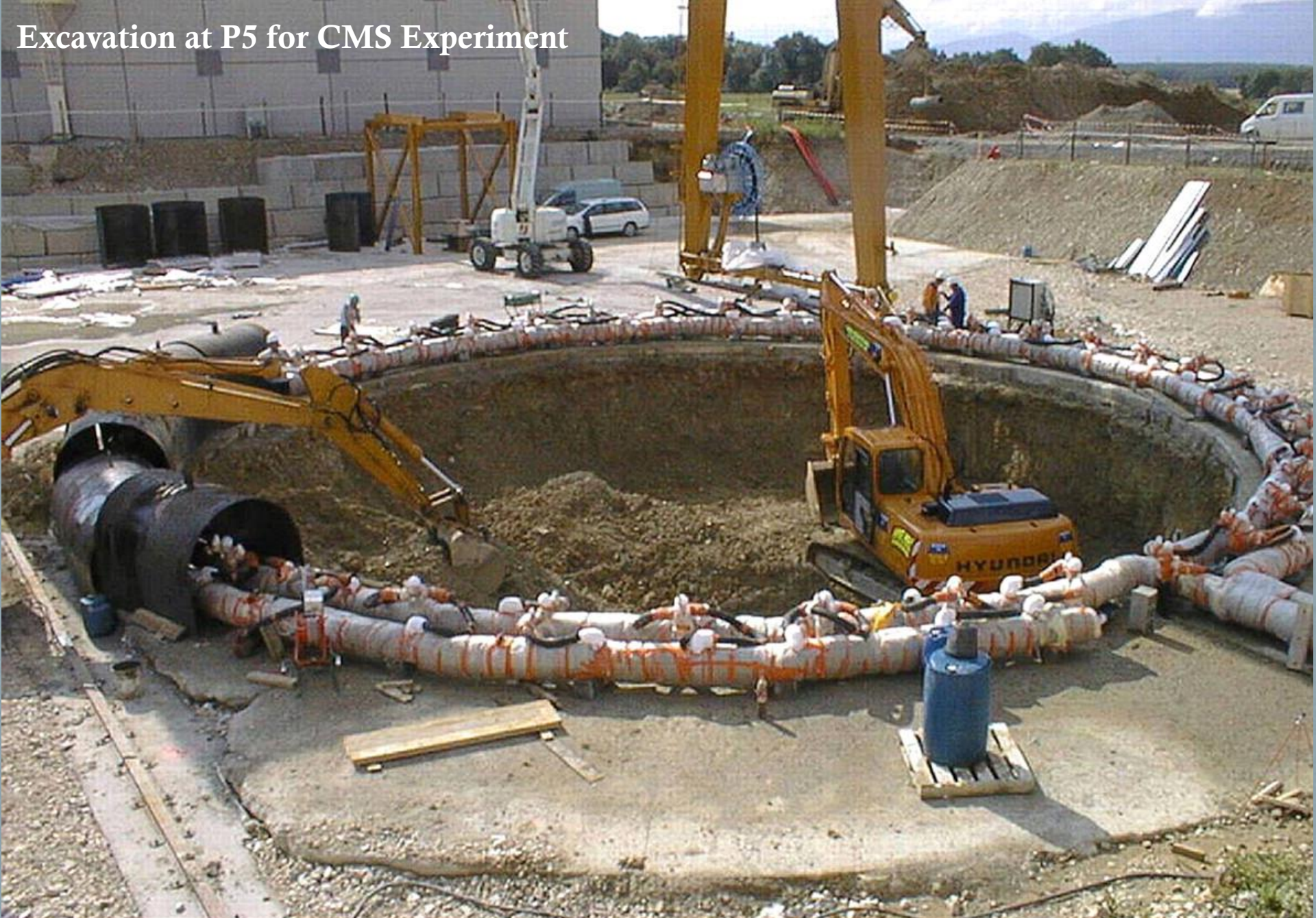
point 5-excavation commencement of PM54 shaft — 09 Jul 1999 CERN ST-CE
