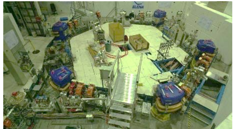
ELENA ring magnets installation in progress
