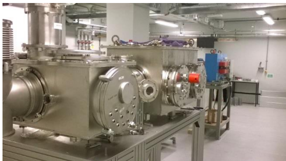
ALPHA-X beam line installation nearing completion in Bunker C
