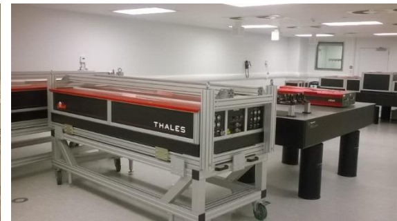
350TW laser installation underway in clean room
