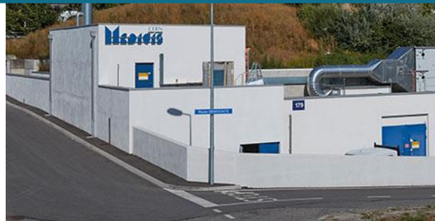
Building delivered 15 Oct. 2014
