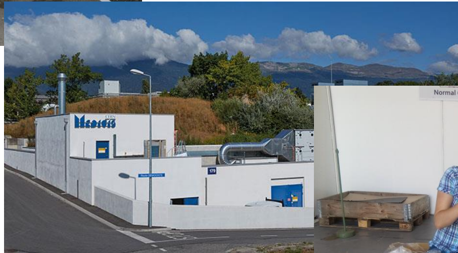
Building delivered 15 Oct. 2014
