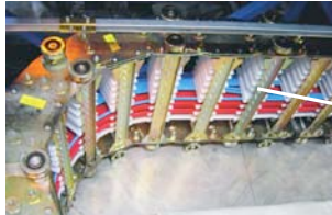
LAr flexible lines during installation, now completed
