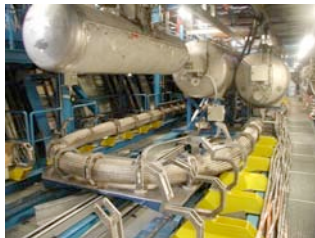
LAr flexible lines during installation, now completed
