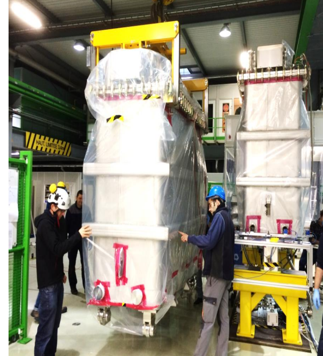
Co-activity CM1 refurbishment / CM2 final testing at SM18
