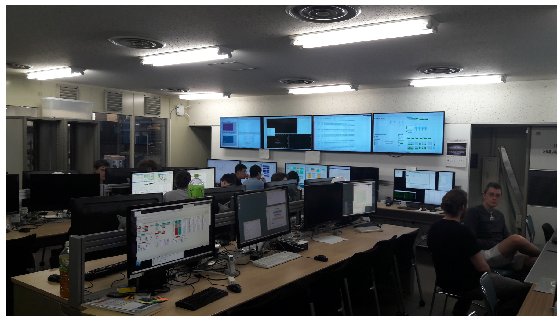
Figure 1: Belle II control room.
