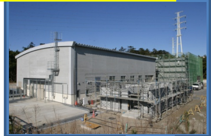
Neutrino monitor building
