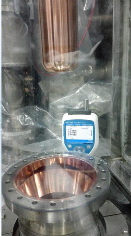
New window waiting for put down: particle measuring
