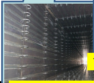
Decay volume completed
