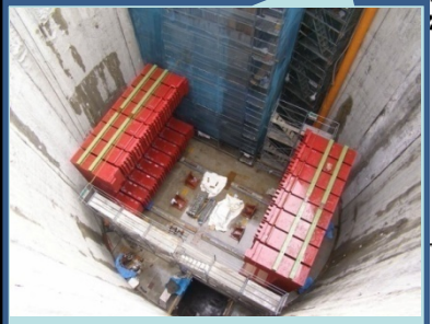
Refurbished UA1 magnet installed
