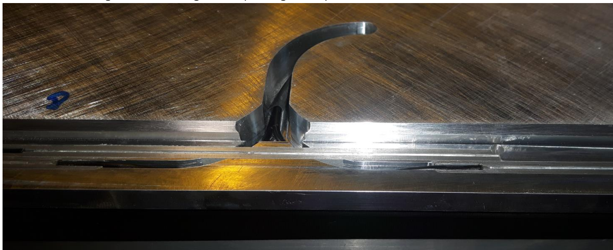
Figure 20 Crossing of cables and light bars
