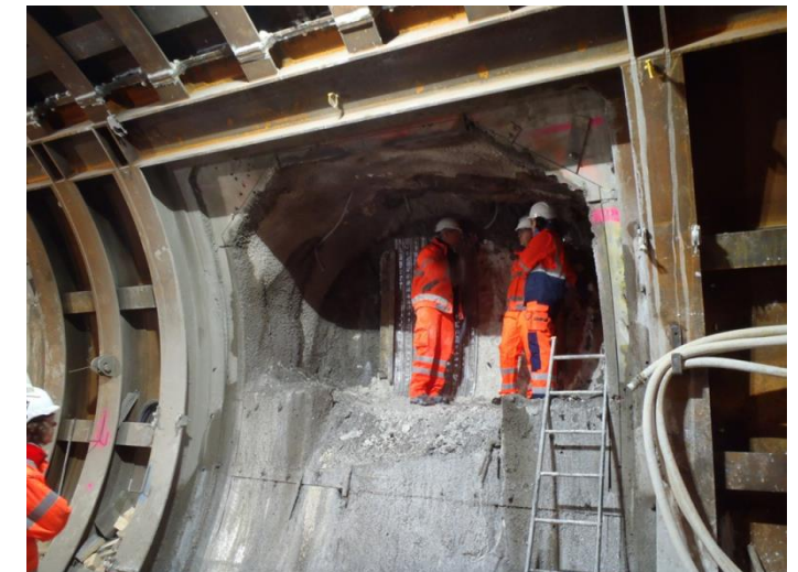
Crossrail – Cross Passage Temporary Frames
