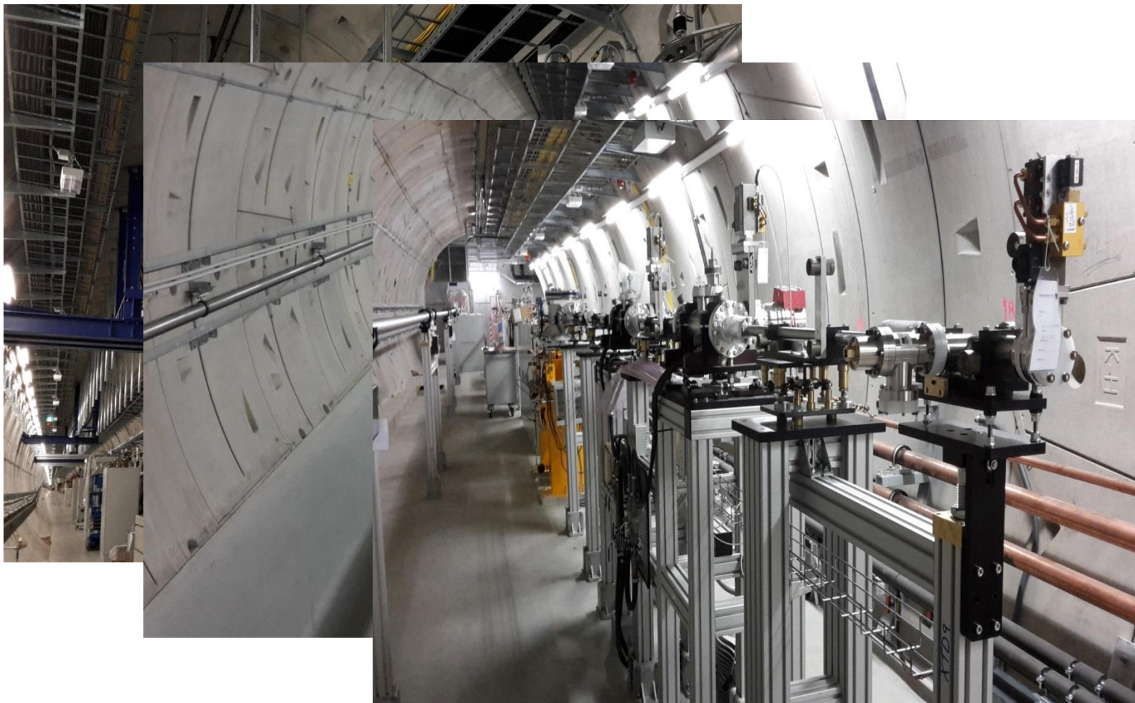
Differential pump + XGM in XTD9
