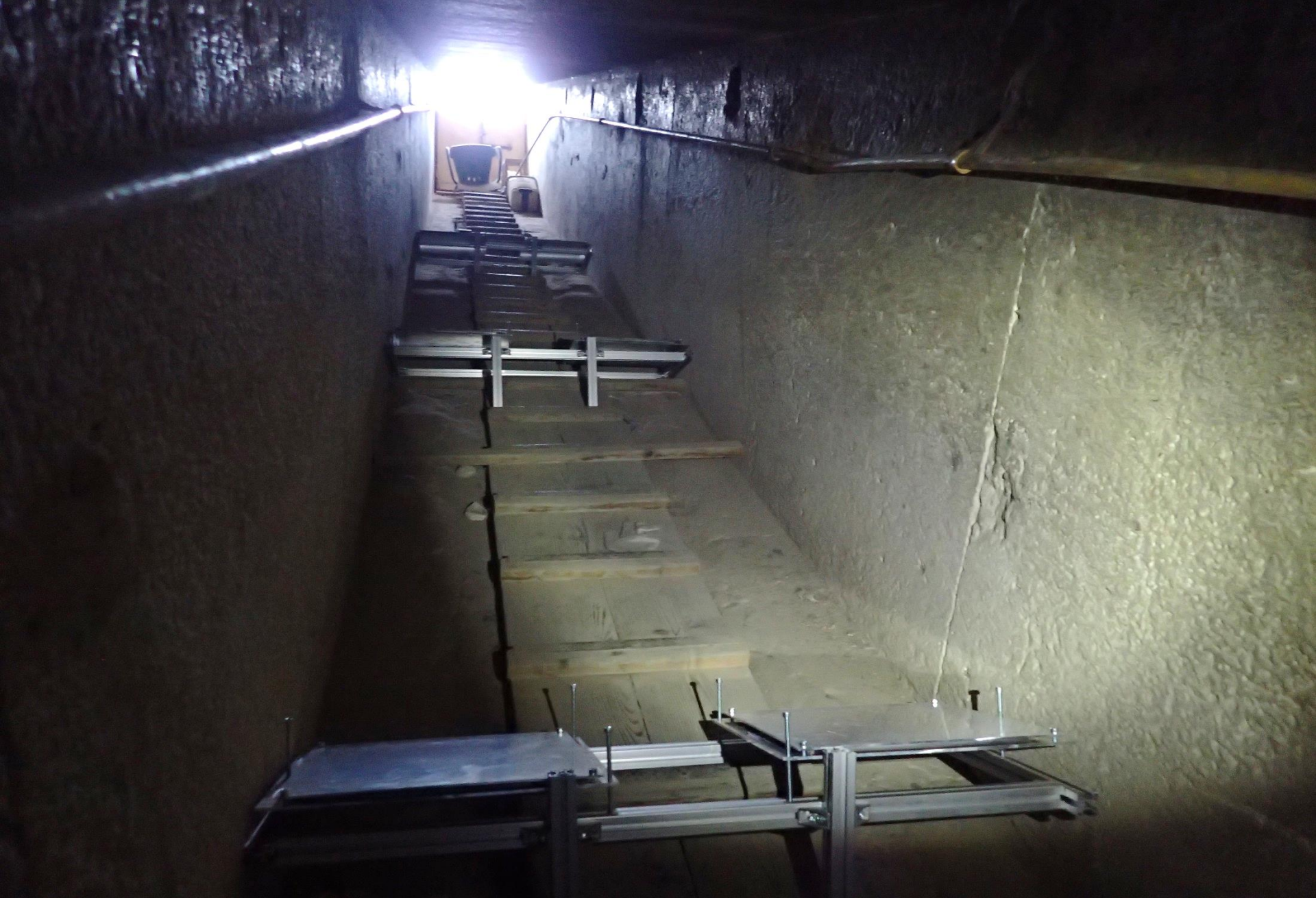
Additional measurement in Descending Corridor
