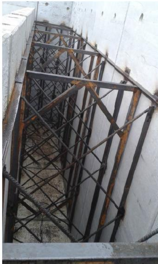
Space between the wall panels
