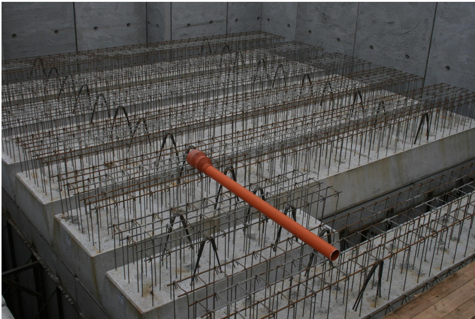
Installed slab plates ready for concreting
