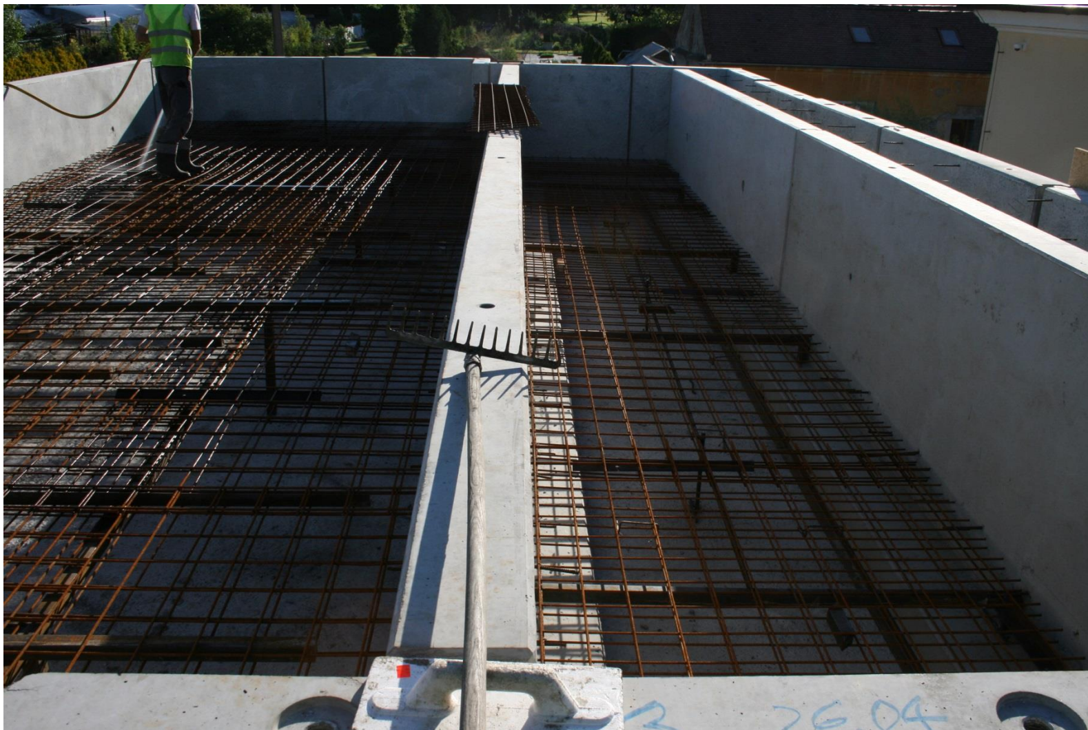
Preparation for final concreting of the ceiling slab
