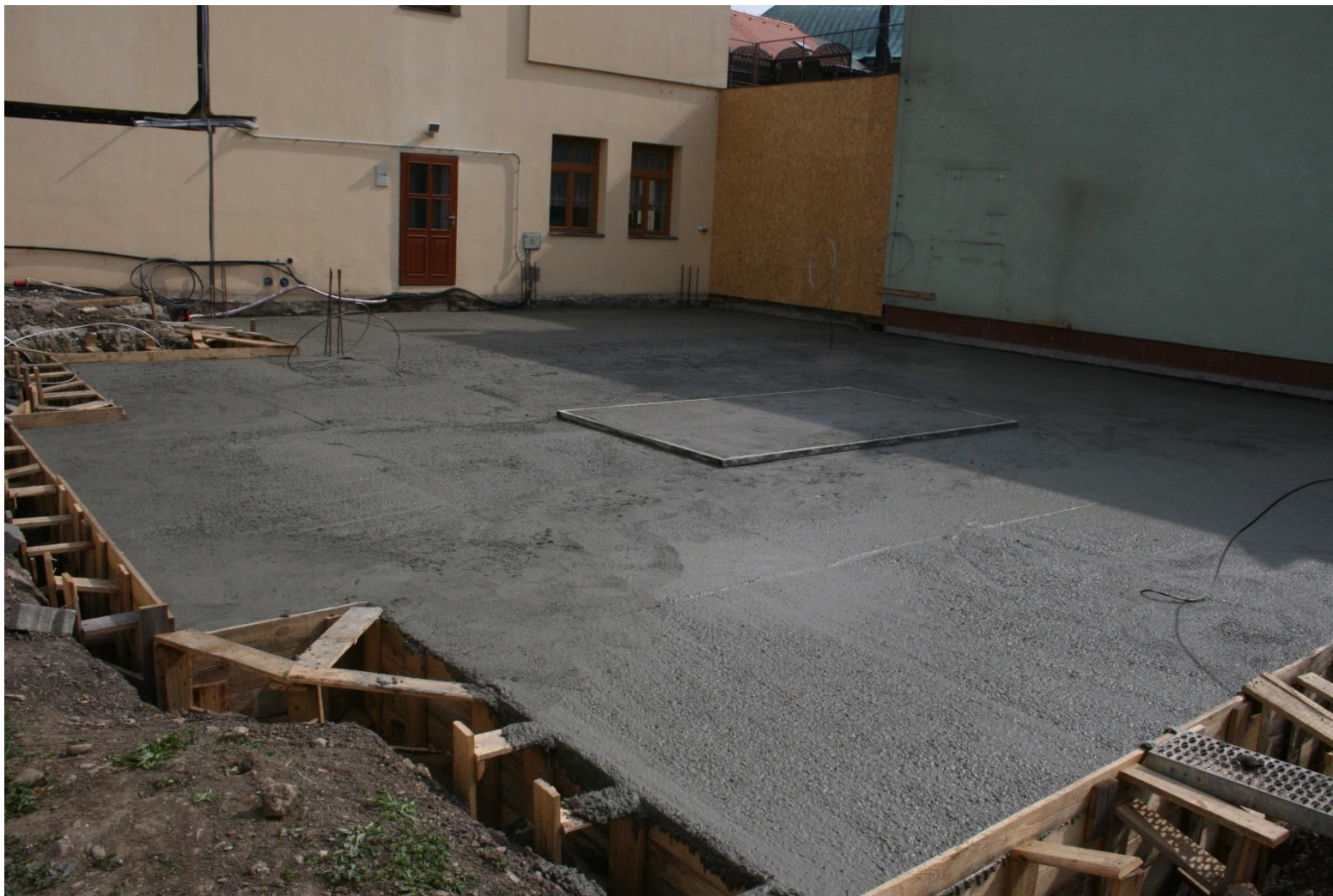
The foundation slab after concreting
