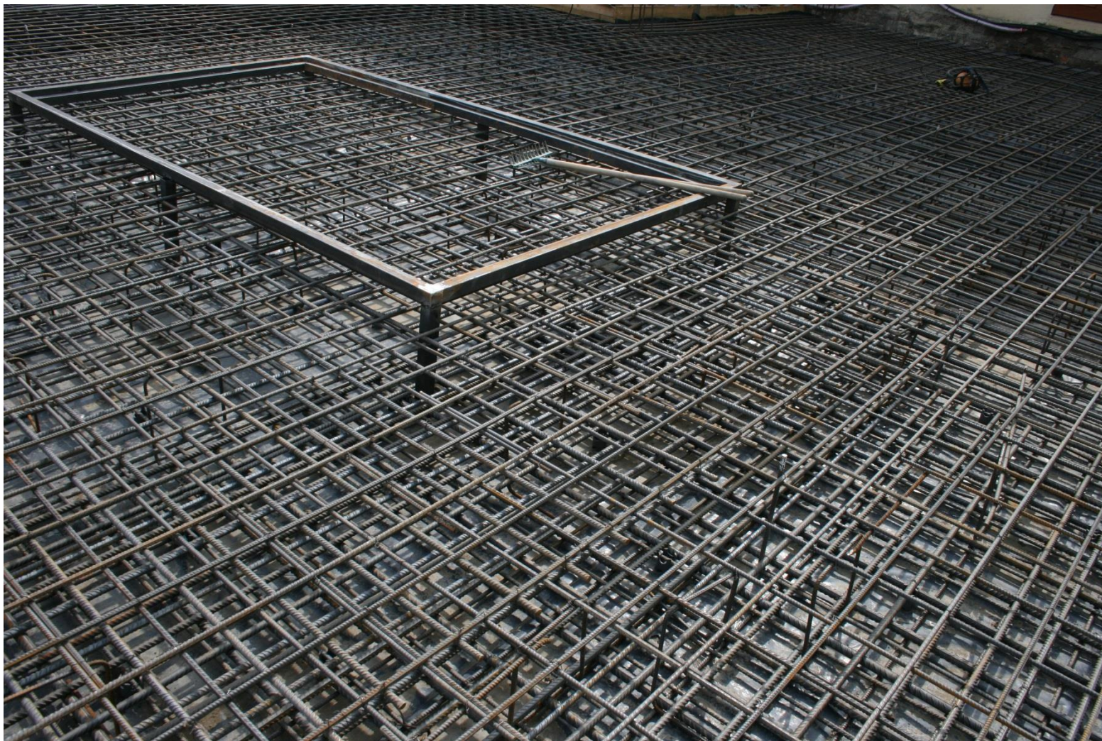
Reinforcement of the foundation slab
