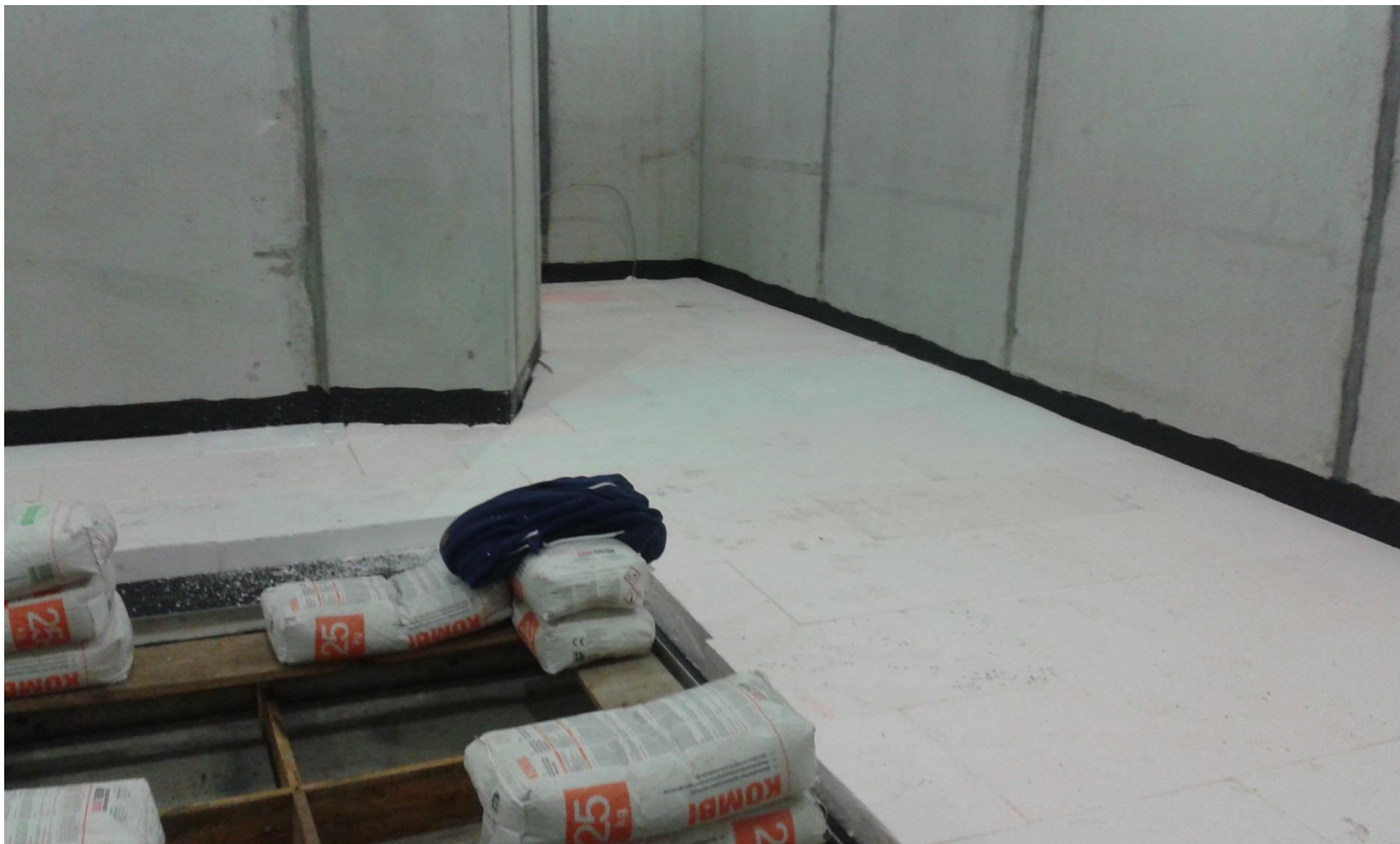
Preparation for floor screeding
