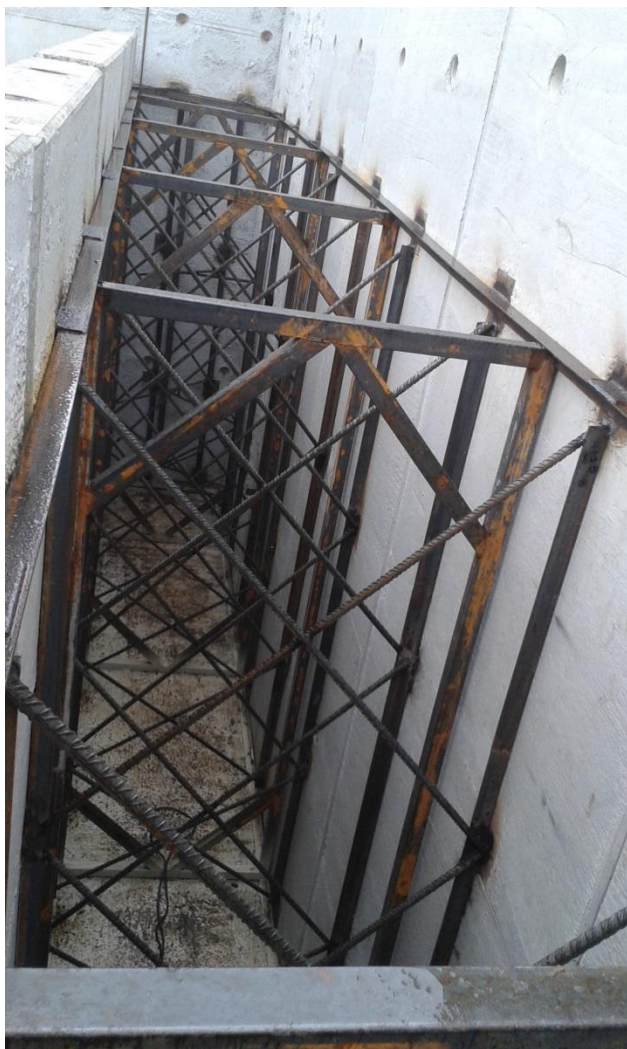
Space between the wall panels
