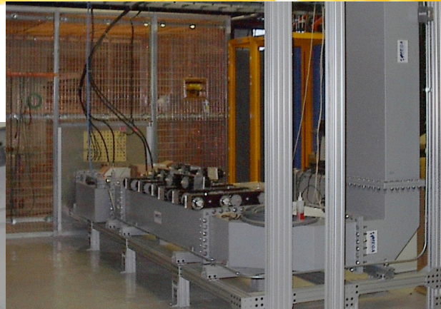
RF component test cage up to 2.5 MW
