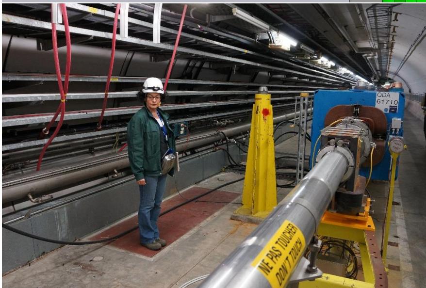
Figure 3: Red steel cover, for inspection during the coming TS
