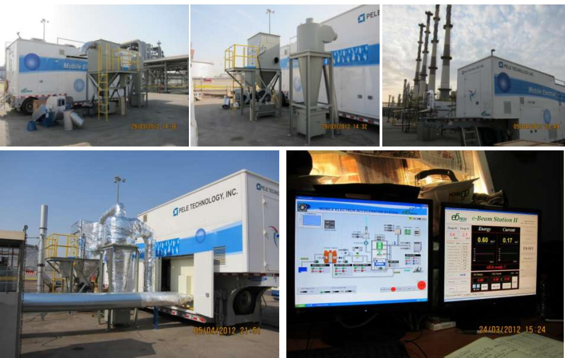
Mobile e-beam in Flue gas Purification from oil-refinery in Saudi Arabia
