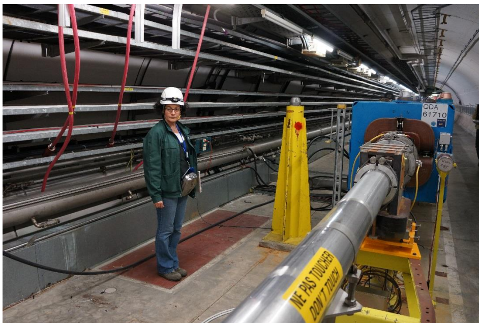
Figure 3 – Red steel plate at the floor in 617, to be inspected during the September TS
