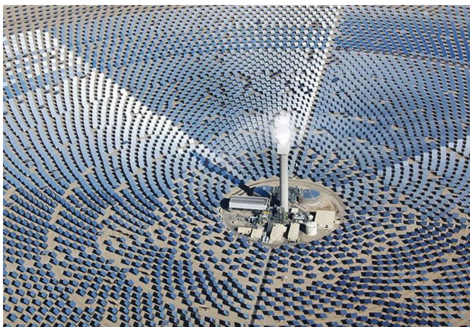
Crescent Dunes CSP power plant, Tonopah, Nevada
