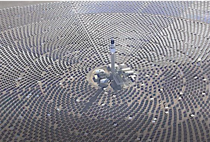
Crescent Dunes CSP power plant, Tonopah, Nevada
