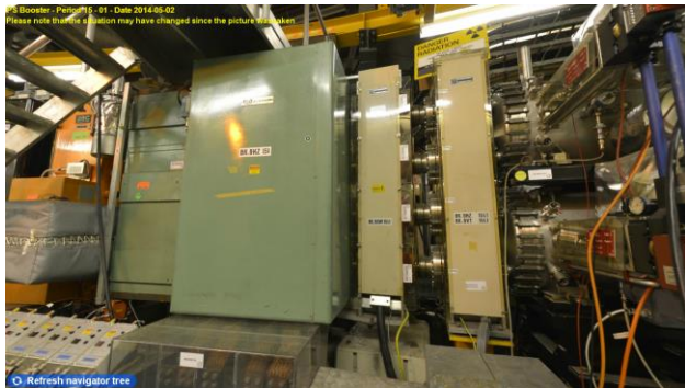
Example of activity: BHZ151 vacuum chamber consolidation
