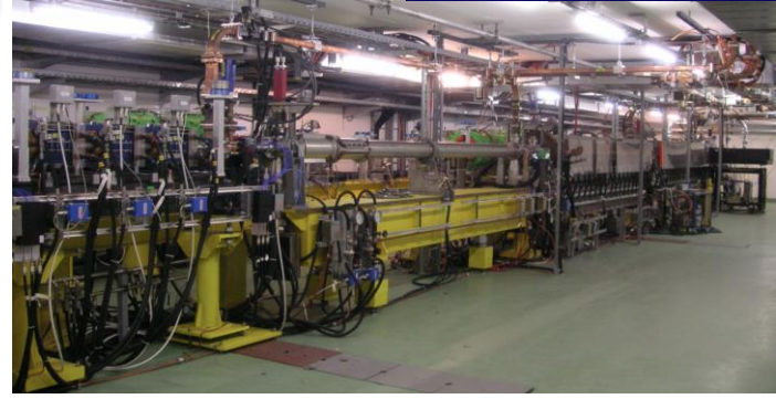
Probe Beam Linac : CALIFES S-band linac, with RF-gun. Fits entirely inside the CLEX room.
