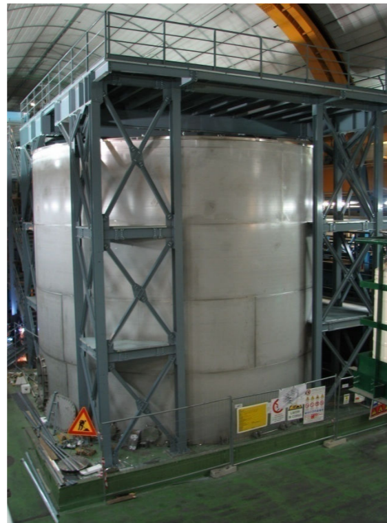
Water tank (July 2008)
